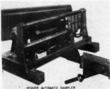
DENVER AUTOMATIC SAMPLER
